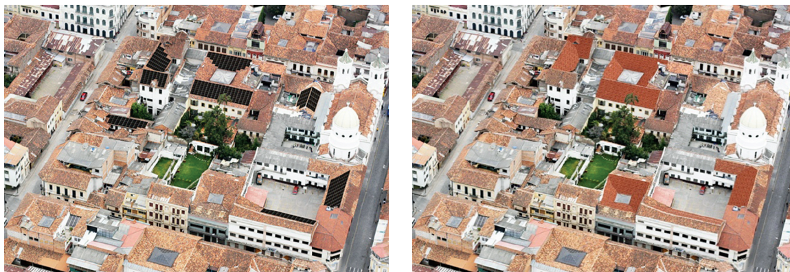
FIGURE 13. (a) Photo of PV roof tiles on rooftops; (b) Photo of 60-cell silica panels on roofs
